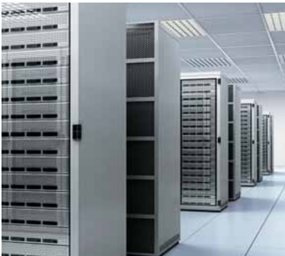
POWER MANAGEMENT & MULTIMARKET
